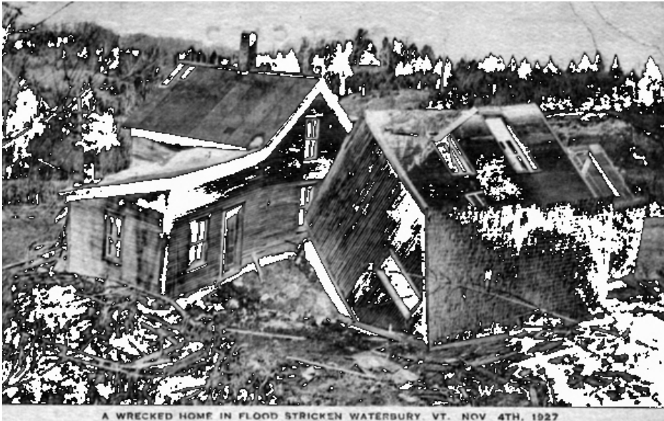
A WRECKED HOME IN FLOOD STRICKEN WATERBURY, VT. NOV. 4TH, 1927
